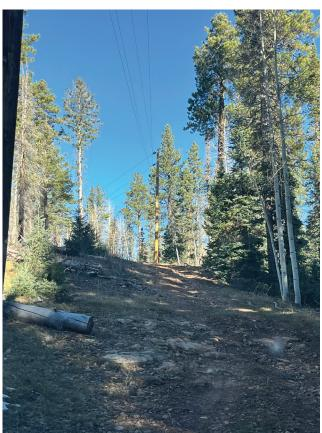
The proposed project consists of replacing a portion of an existing 25 kV overhead 3-phase power line with a underground line to mitigate the risk to and from wildland fire.
