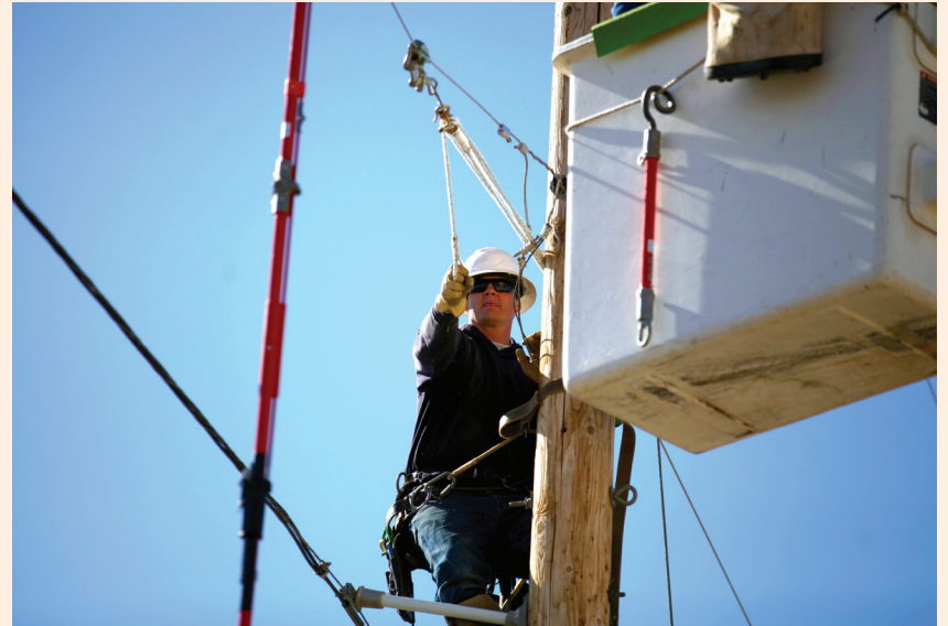
Tyler Gates works on a line on Hwy 89 in Kanab.
