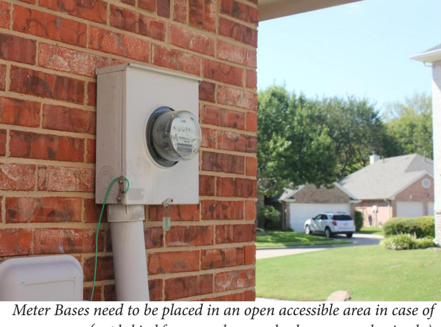
*Meter Bases need to be placed in an open accessible area in case of emergency. (not behind fences, enclosures, shrubs, or around animals.)*
