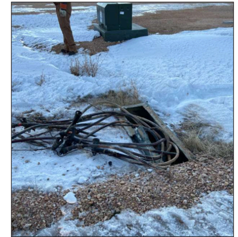
These Garkane transformers were hit by vehicles, knocking them off their pedestals, leaving deadly high voltage lines exposed. (352100) Luckily no one was hurt in either incident, but could've been deadly.
