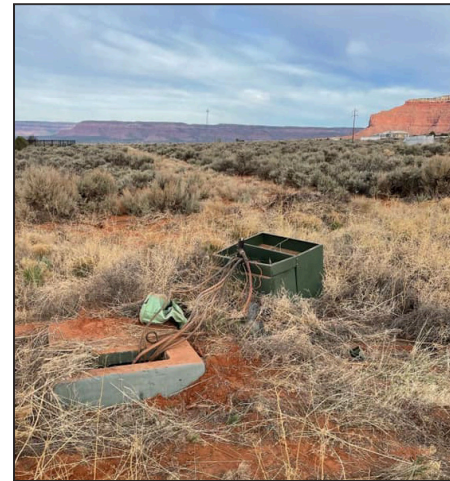
These Garkane transformers were hit by vehicles, knocking them off their pedestals, leaving deadly high voltage lines exposed. (352100) Luckily no one was hurt in either incident, but could've been deadly.
