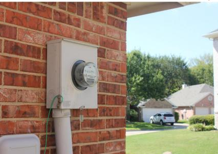
Meter Bases need to be placed in an open accessible area in case of emergency. (not behind fences, enclosures, shrubs, or around animals.)
